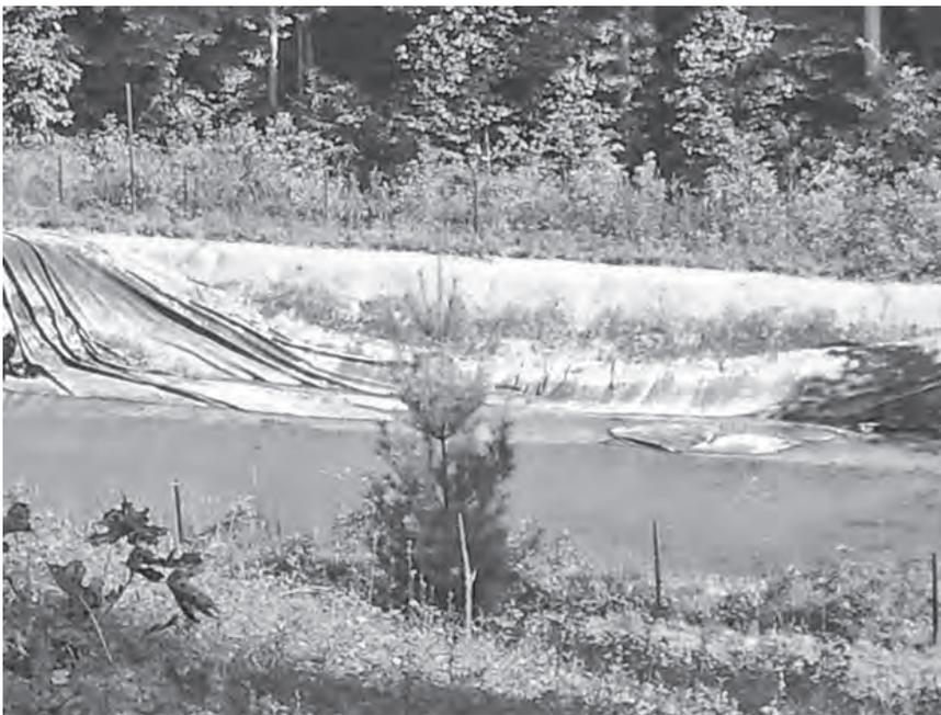
Picture taken in response to WVDEP claims that dye tests were performed and the pits in Lochgelly were not leaking. Notice the "high water" mark is about the pit liner. See [www.dirtysecretwater.com](http://www.dirtysecretwater.com) for color graphic.
